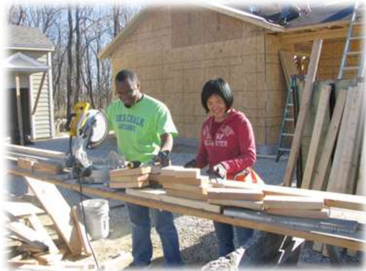
David and Ying working on the build site, Dec. 2012
